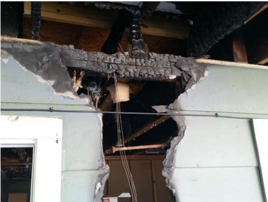
Fire damage on Unit #201
