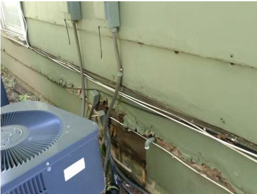
North side of Building #4, note damaged siding
