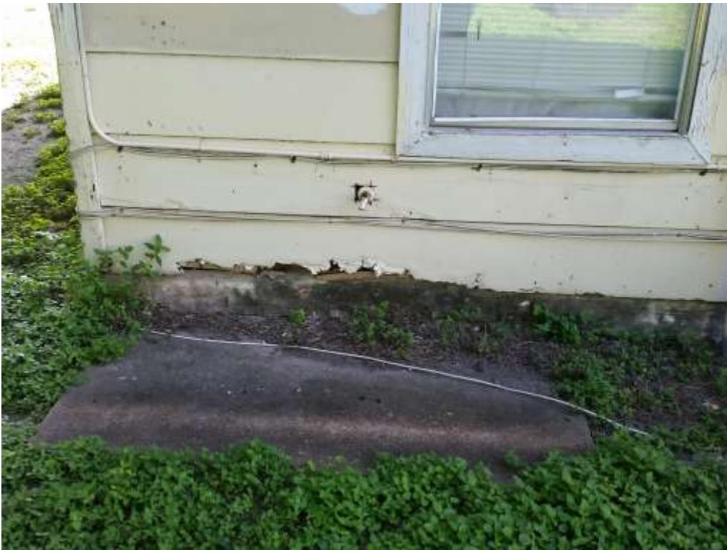
West side of Building #3, note damaged siding
